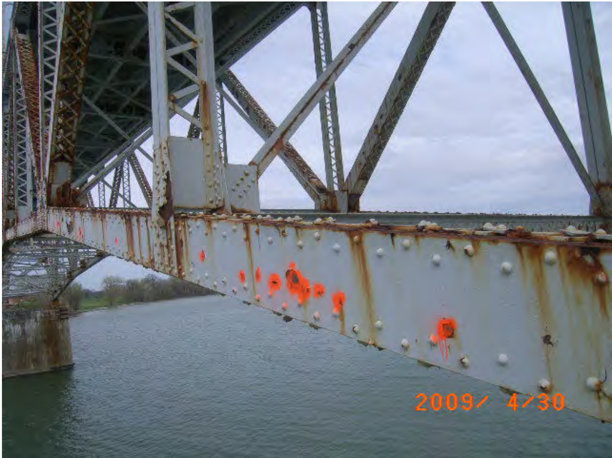
Figure 121. Span 6 lower chord at L00-L02.
