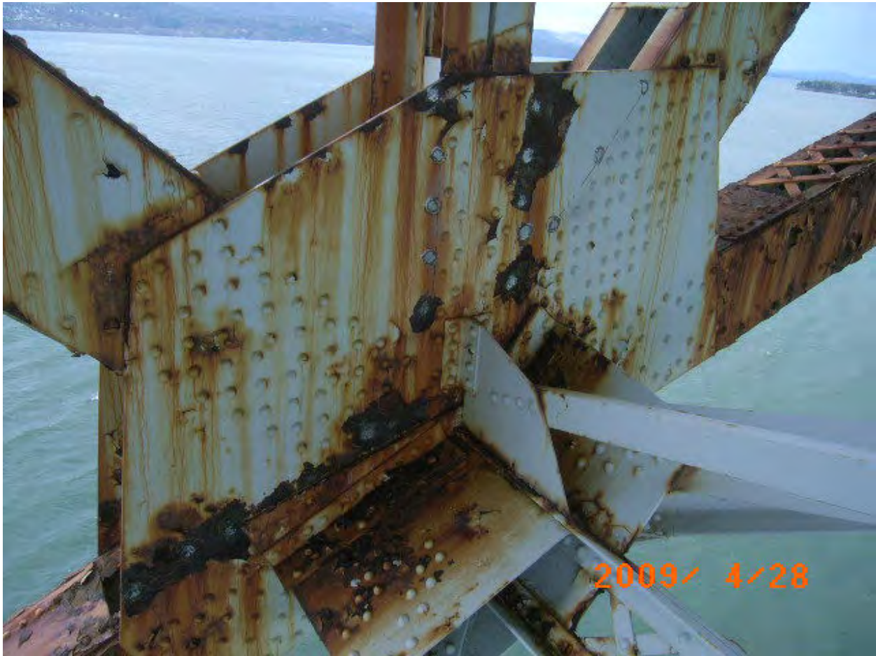
Figure 115. Span 7 lower chord connection at L12, interior side.
