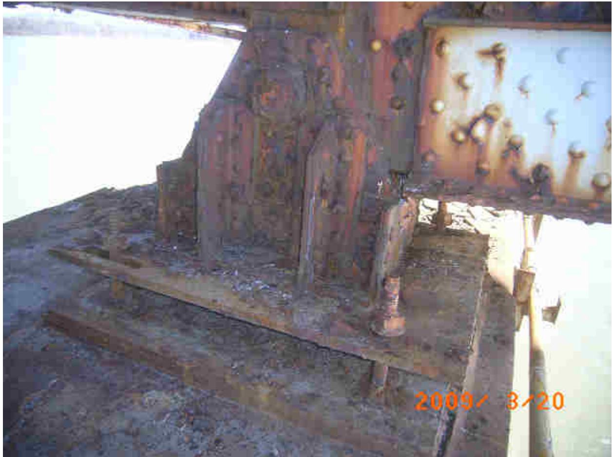
Figure 126. Span 5 at Pier 5, right truss roller bearing.
