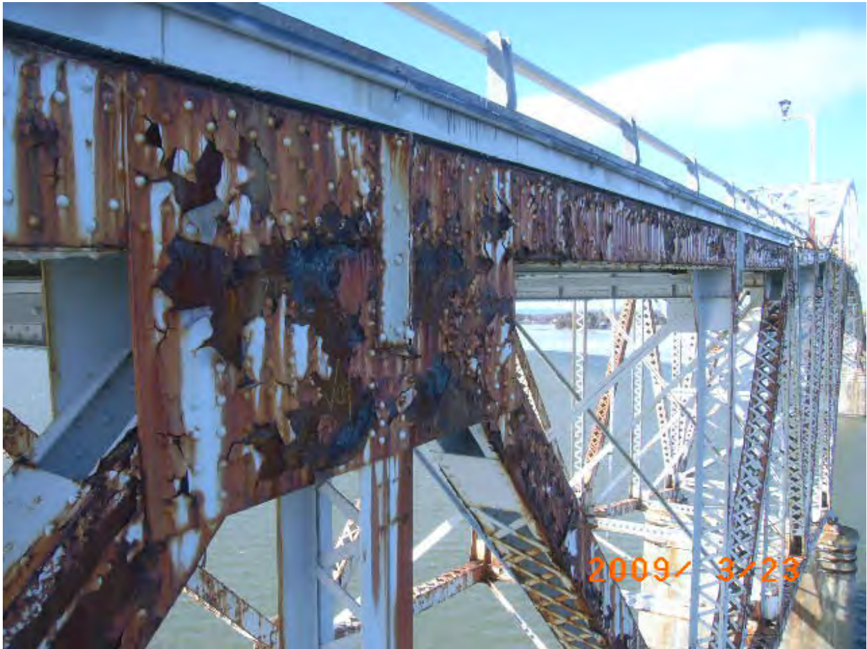
Figure 119. Span 6 upper chord connection at U05.
