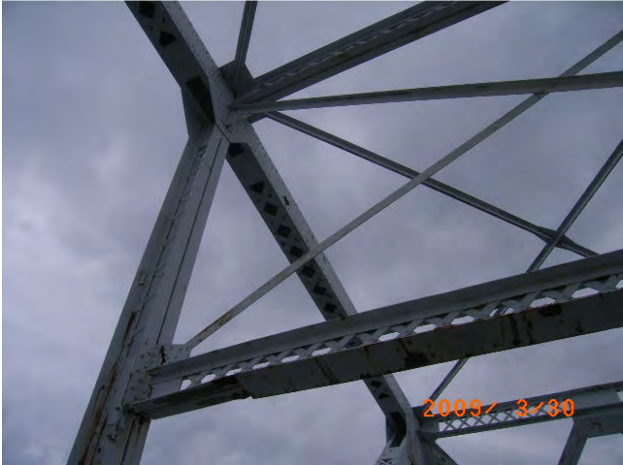
Figure 111. Span 7 strut, upper chord, and sway bracing at Panel Point 16.
