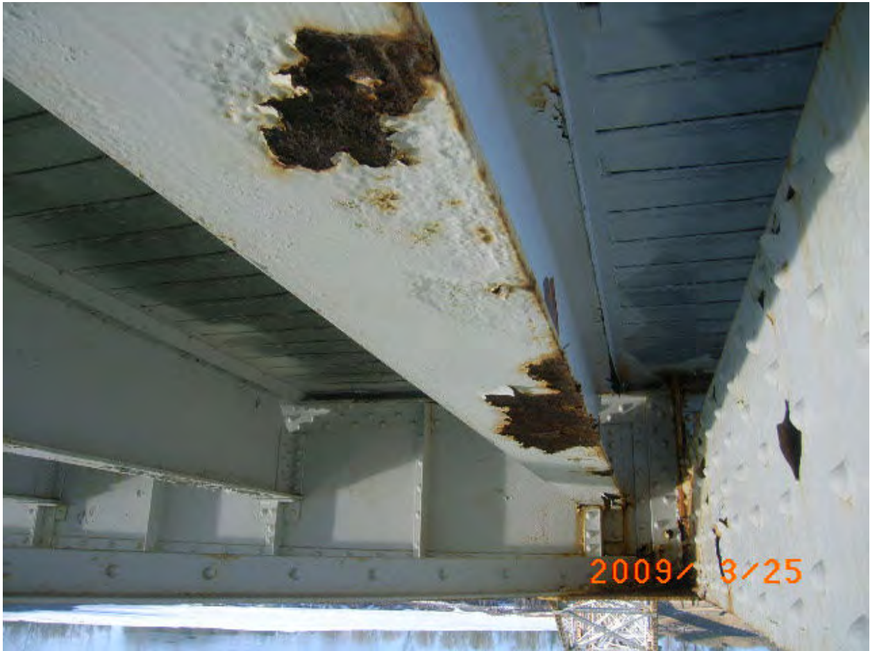
Figure 118. Span 7 Panel 20 stringer.
