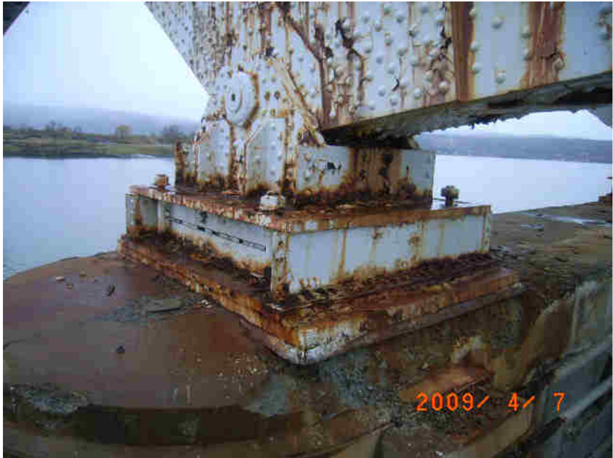
Figure 128. Spans 7/8 at Pier 7, right truss rocker bearing.
