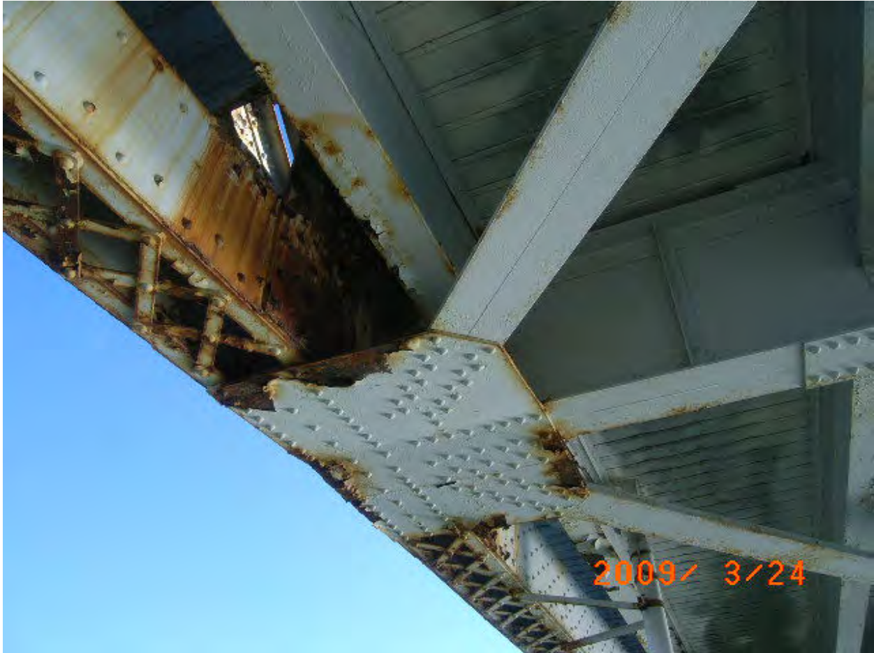
Figure 116. Span 7 lower chord lateral connection at L14.
