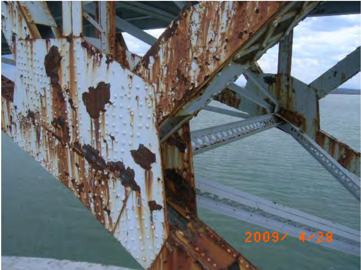
Figure 114. Span 7, lower chord connection at L12.
