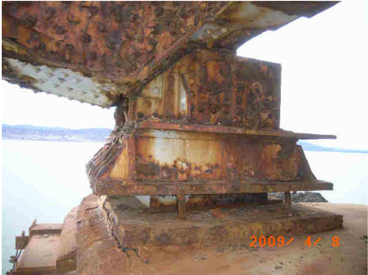
Figure 129. Span 8 at Pier 8, left truss roller bearing.
