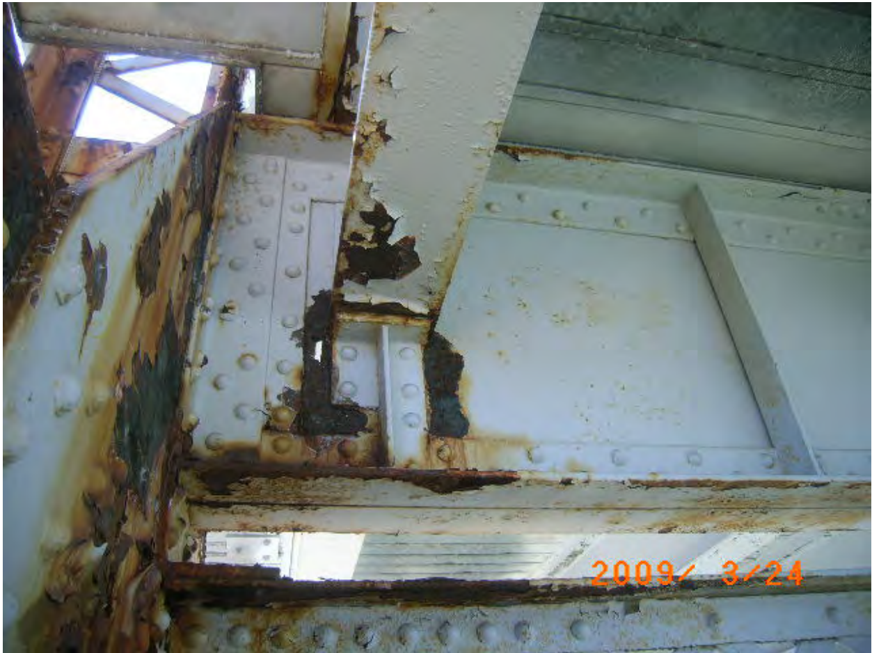
Figure 117. Span 7 Floor Beam 13.
