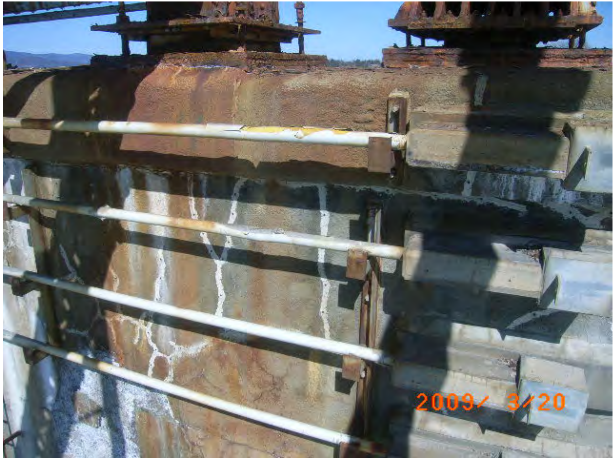
Figure 131. Pier 5 upper south side of stem, cap and tensioners.
