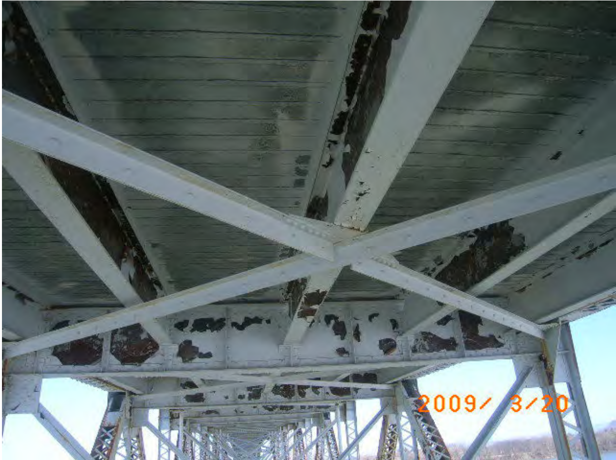
Figure 123. Span 6, Panel 2, laterals, stringers, and floor beam (Spans 4, 5, 6, 8, 9 are similar).
