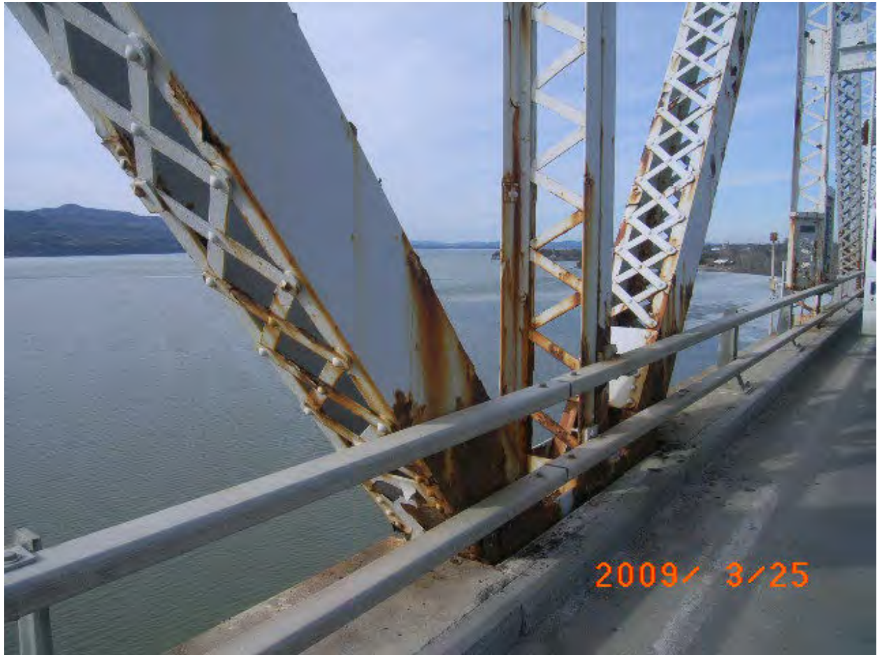
Figure 112. Span 7 deck at connection L16.
